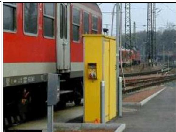
*Another example of compact structure of the water tanking and sewage removal station with the external installation option. Source: <http://www.vogelsang.info/?id=30>*
