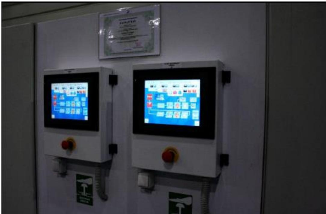
*Visualisation of the control system on the screens controlling the pre-paint treatment station and the paint facility (Photo: Nova VERTA)*
