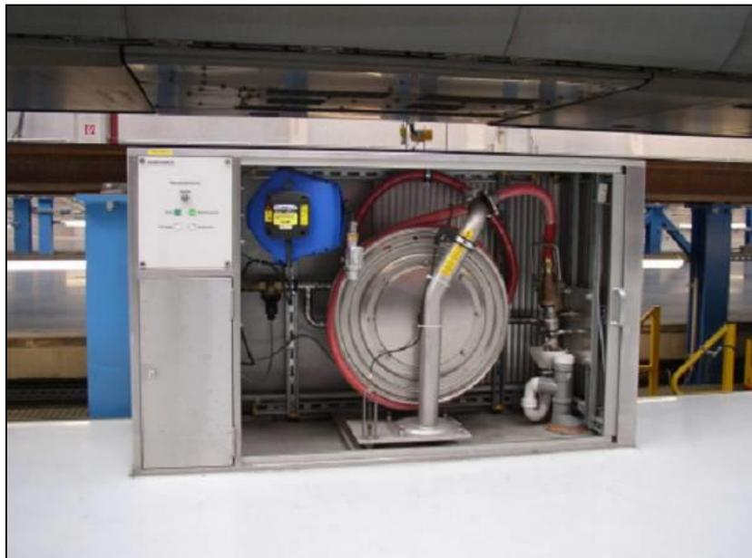
*Example of compact structure of the water tanking and sewage removal station.*
